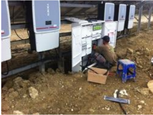
Inverter Installation
